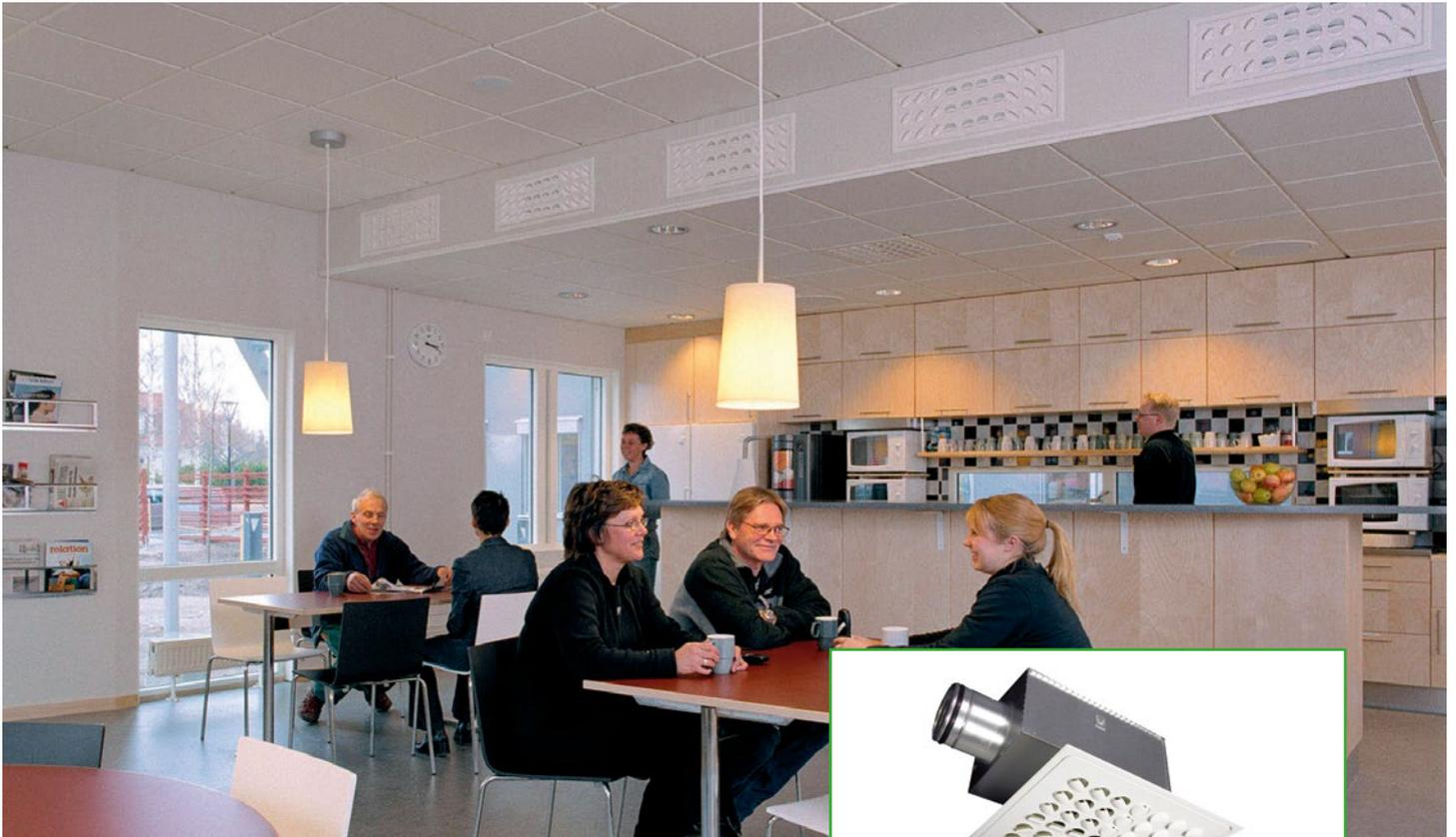
Even cool air can be supplied into a room without draught when Swegon's disc diffusers are used. Fresh air is effectively mixed into the warm air in the room, thus providing more comfortable air exchange. Swegon's unique, aerodynamically designed discs always make it possible to set the diffusion pattern so that no one will have to feel a cold draught in the room. The diffusion pattern is very simple to alter any time without affecting the sound level, airflow or pressure!
