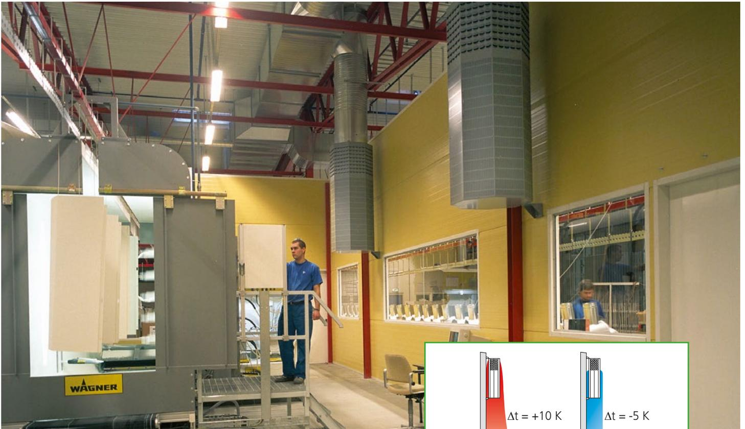
The Booster is a unique air diffuser because it can alternate displacement ventilation. The air diffuser is designed for use in buildings with high ceilings (e.g. sports centres, shopping centres, factories, etc.) and can be either installed suspended from the ceiling or secured to a wall. In this way, the Booster doesn't take up any floor space.
