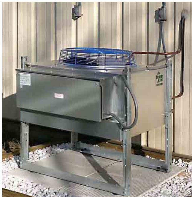
Remote Outdoor Condenser (ROC) piped to unit located inside facility.
