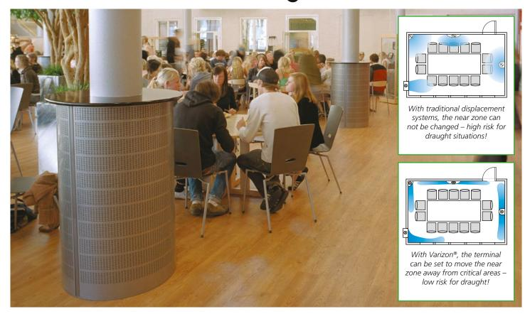
Swegon's displacement terminals are made to effectively discharge air at low velocity. To ensure good comfort in rooms, most of the air terminal devices are equipped with Swegon's flexible Varizon® air distribution system, which makes it possible to alter the diffusion pattern. In rooms with high ceilings, substantial energy savings are possible by installing Swegon's displacement terminals with Varizon®.
