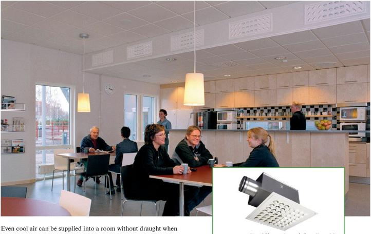
Even cool air can be supplied into a room without draught when Swegon's disc diffusers are used. Fresh air is effectively mixed into the warm air in the room, thus providing more comfortable air exchange. Swegon's unique, aerodynamically designed discs always make it possible to set the diffusion pattern so that no one will have to feel a cold draught in the room. The diffusion pattern is very simple to alter any time without affecting the sound level, airflow or pressure!
