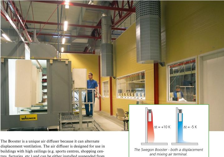
tres, factories, etc.) and can be either installed suspended from the ceiling or secured to a wall. In this way, the Booster doesn't take up any floor space.
